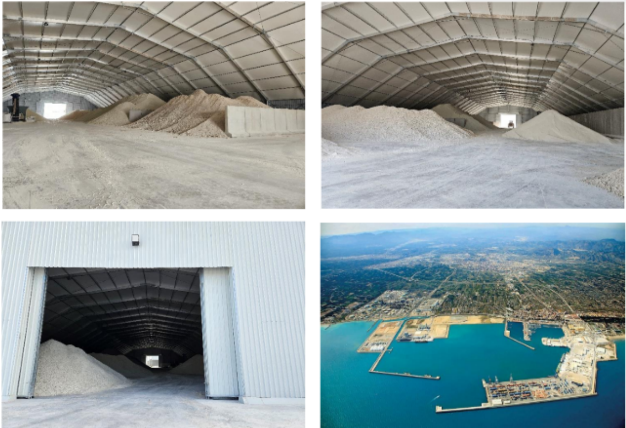
Figure 3: IberoClays warehousing infrastructure at Port of Castellon in Spain
